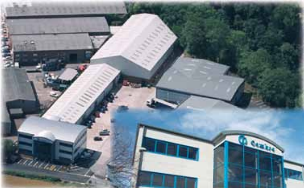
Cembre Ltd. factory in Curdworth (Birmingham)
